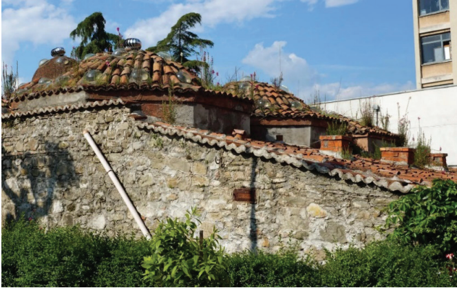
Figure 8: Fortress bathhouse ( hamam ).
